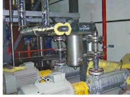
Boiler feed unit with thermosysphon cooling
